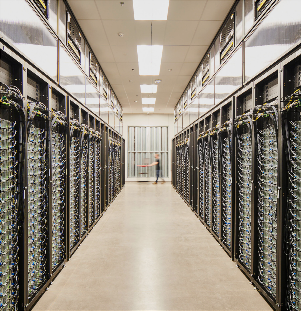
Apple's Reno data center, opened in 2012, takes advantage of the mild climate by cooling its servers with outside air whenever possible.
